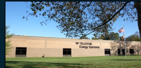
TESI Sparks Facility Sparks, MD
