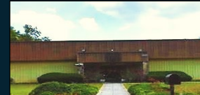
TBE Test and Demonstration Facility Oak Ridge, TN
